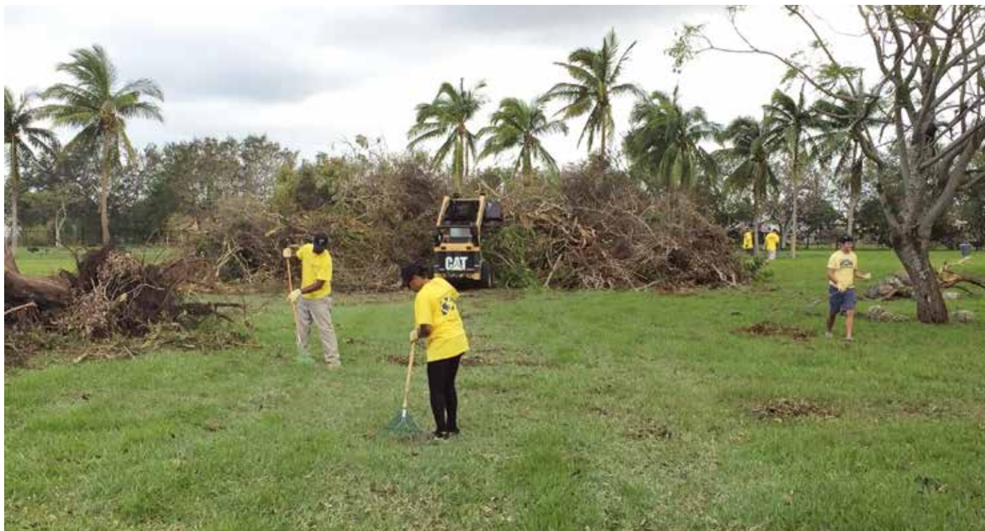
After Hurricane Irma, crews cleared 20 miles of roadways and right-of-ways.
